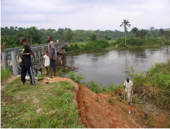
Before Bridge foundation stabilization
