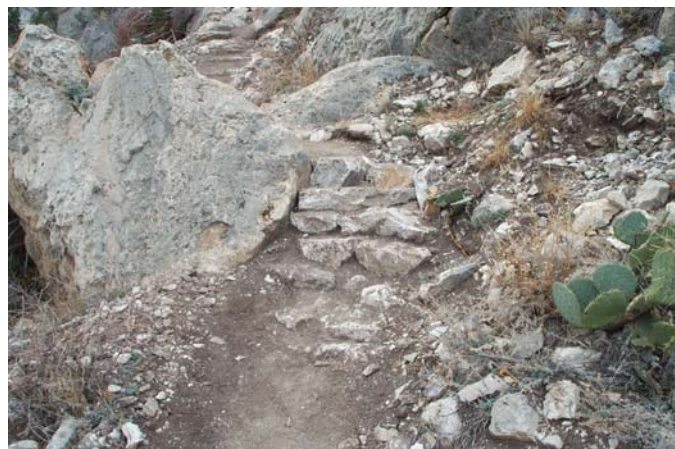
AFTER PHOTO: The trail is now a well-defined path with a stairway in this location. (NPS Photo by Jeff Doryland)
