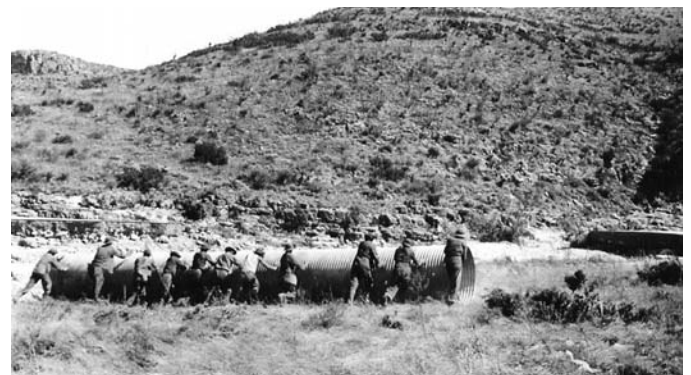
CCC workers installing large culverts along the park road. (NPS Photo)
