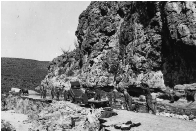
CCC workers repairing the flood-damaged park road in September 1941. (NPS Photo)
