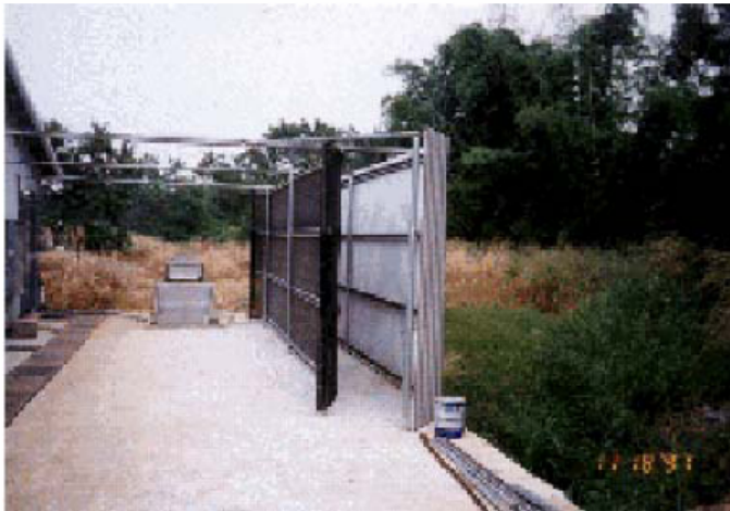
Figure 9. Relevant design considerations and low-cost designs using UV-resistant tarpaulin or plastic material, roofing, or wood fastened to anchored pipe frames or posts are potential options for windbreak walls.
