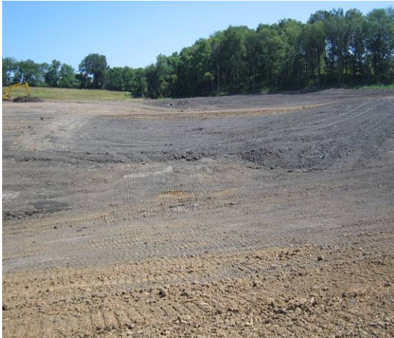
Figure 3. Pond being reconstructed.
