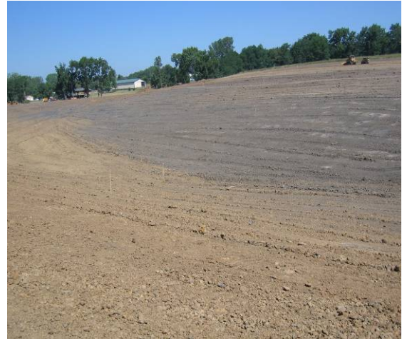
Figure 4. Pond and terraces being reconstructed.
