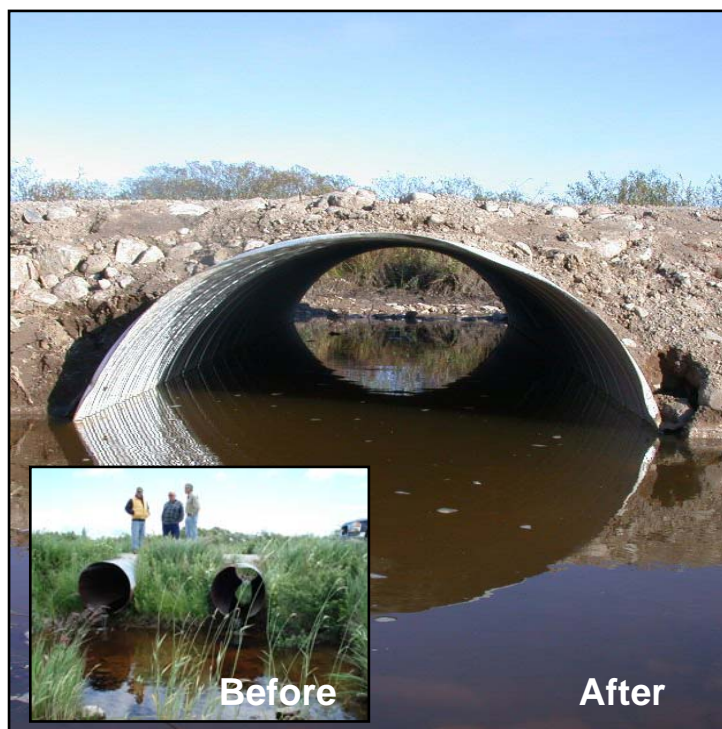
Before: Perched twin culverts on Maxton road crossing of McCormick Creek. Photo: Neal Godby, MDNR. After: The twin culverts were removed and replaced by a single 32-foot long, 8-foot diameter culvert. Photo: Andrea Ania, USFWS.
