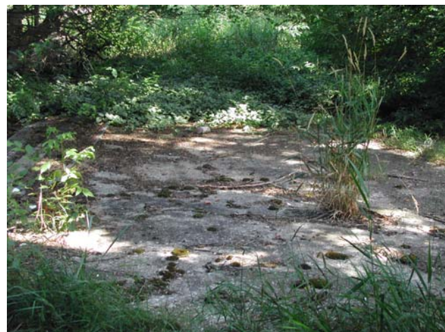
Figure 5. Open area in front of barn entrance
