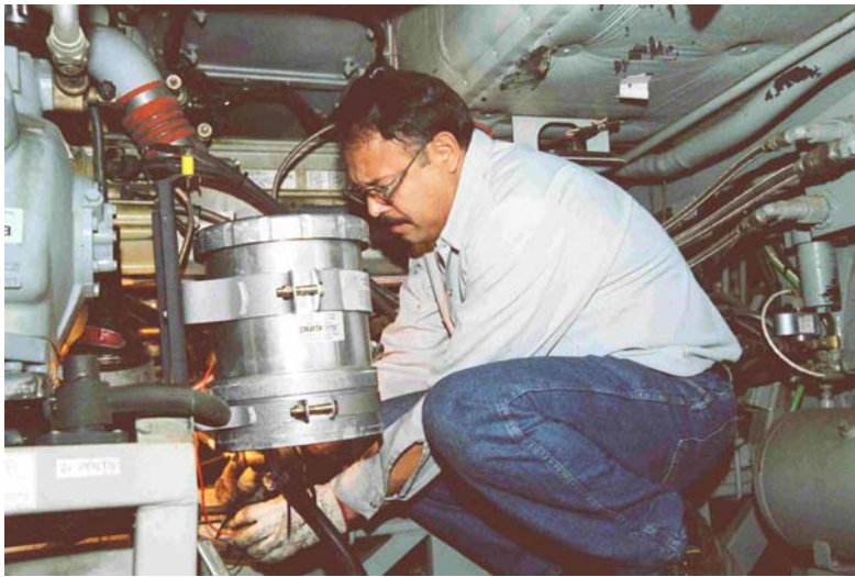
Figure 10. INEEL mechanic installing an oil bypass filter on a bus with a Series 60 Detroit Diesel engine.
