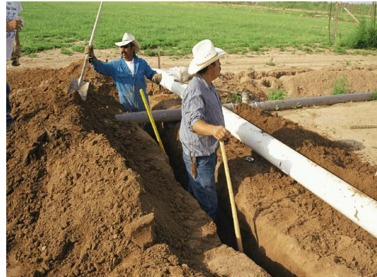
Figure 6. Delivery line installation.
