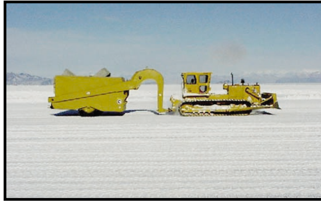
Photo by Gary Cardullo/Special to the Antarctic Sun A D-8 tractor tows a 100-ton roller, compacting the snow on Pegasus runway.
