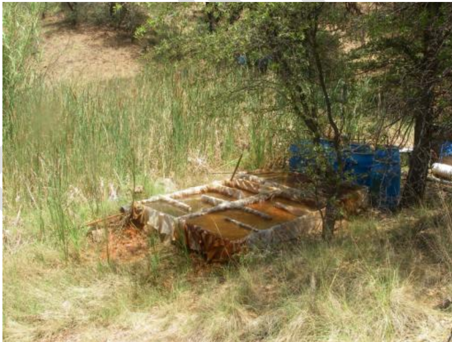
Figure 8. January Adit discharge continuing through treatment system.
