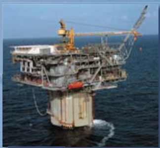
Neptune, the world's first SPAR, is installed in the GOM in 1,851 feet of water
