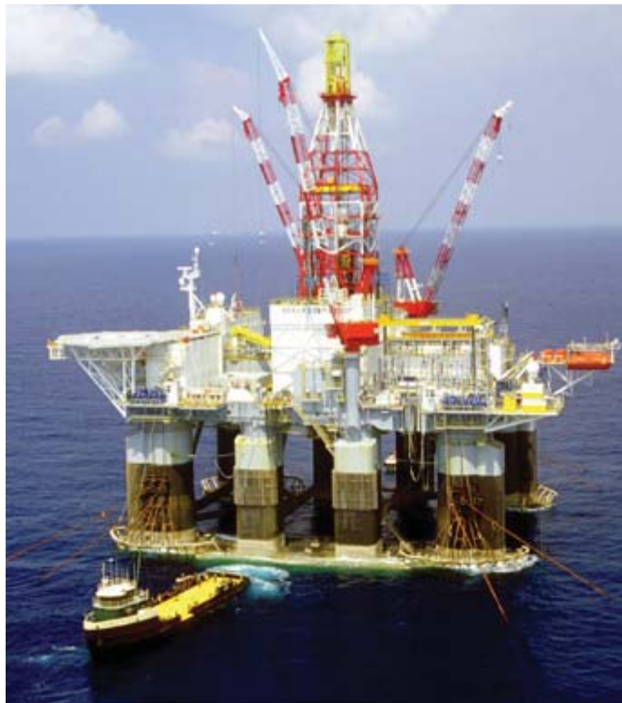
Photo of the production platform Ocean Confidence .
