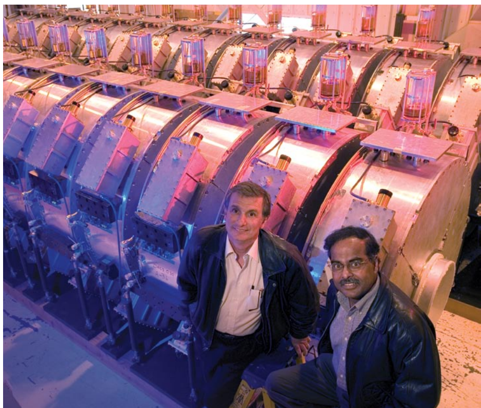
DARHT Project Director Ray Scarpetti (left) and Deputy Director Subrata Nath, standing proudly beside the long rows of refurbished cells now being installed in the second axis.
