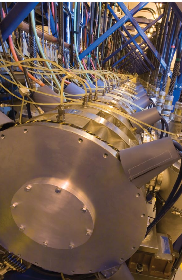
The 3-foot-diameter induction cells of DARHT's first axis.
