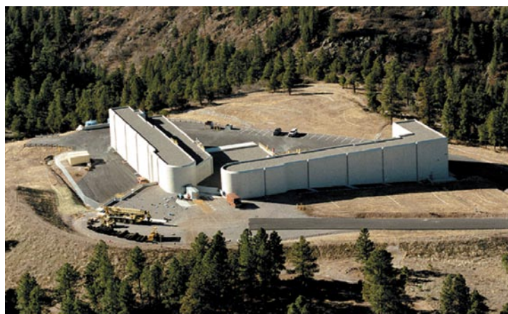
Construction of the twin accelerator buildings for DARHT's two axes began in 1994.
