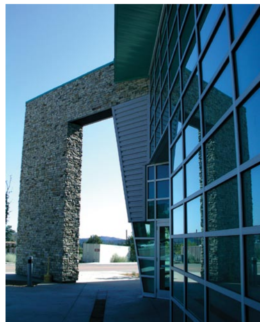
Entrance to the CINT gateway at Los Alamos. The CINT core facility is at Sandia National Laboratories in Albuquerque.
