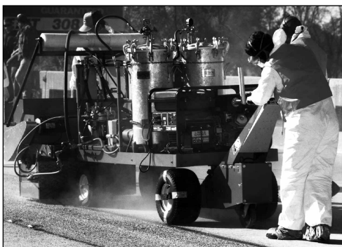
Workers resurface bridge with environmentally friendly spray system.
