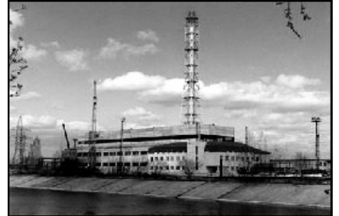
Construction of the Chornobyl replacement heat plant was completed June 2001.
