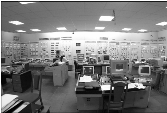
This full-scope simulator was designed to enhance operational safety of the Rivne site's Soviet-designed MWe VVER-1000 Unit 3 reactor.
