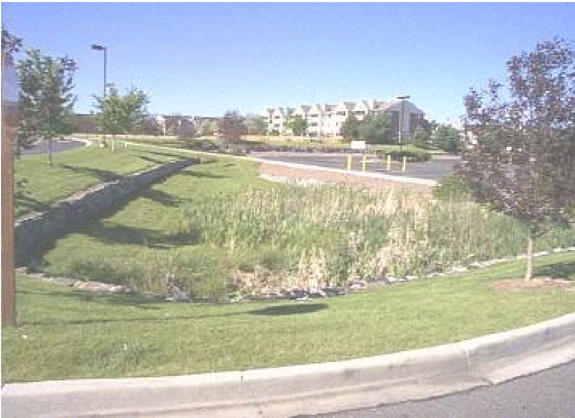
Figure 2-1 Typical Dry Pond (UDFCD, 1999)
