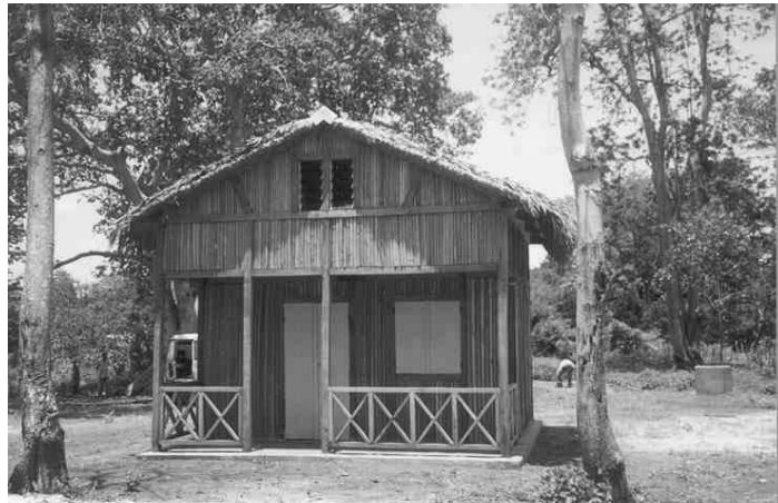
The Andrafiabe village has been quite receptive to manage the cases villageoises constructed by LDI for the Ankarana Mandroso Association
