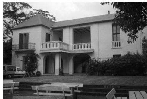
The Fontenay Resort
