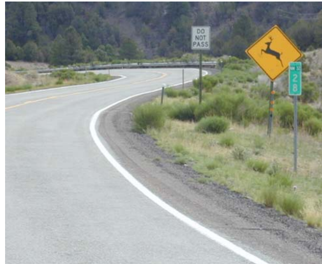
Figure 9. Typical Deer Warning Application
