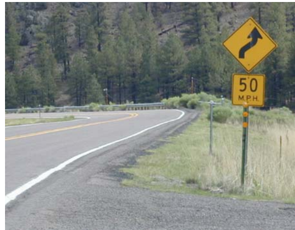
Figure 7. Sign inconsistent with roadway
