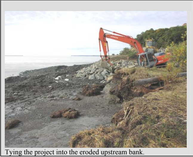
Tying the project into the eroded upstream bank.
