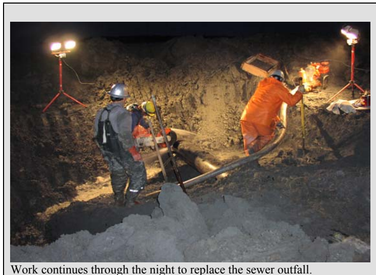
Work continues through the night to replace the sewer outfall.
