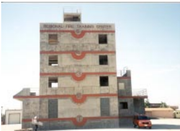
Regional Fire Training Center
