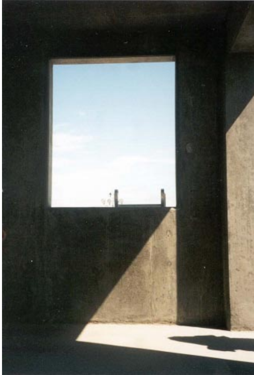
Photo 3. Forty-two-inch Window Sill and Ladder Tip
