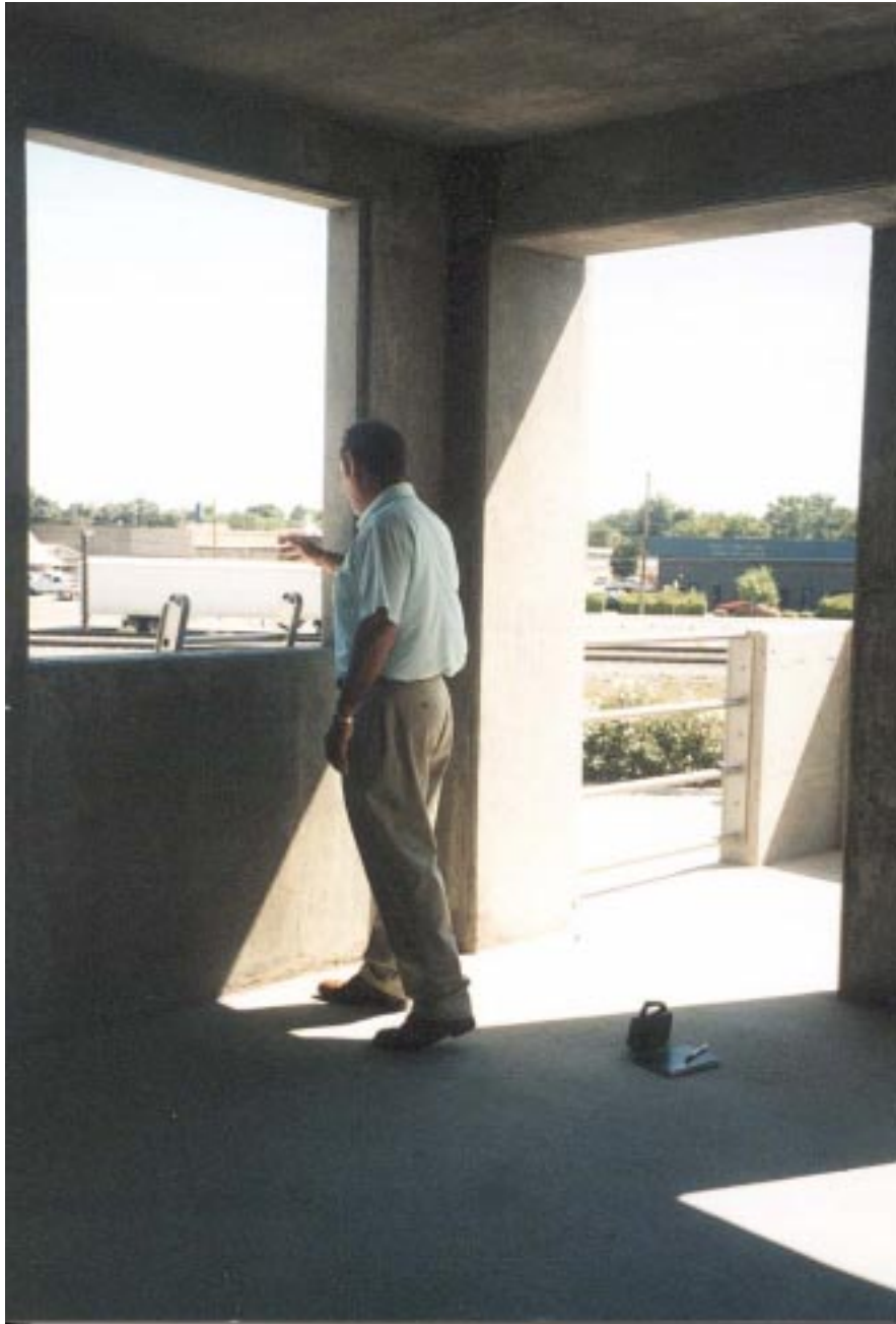
Photo 4. Position of Victim Prior to Incident
