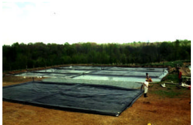
Installation of new cover at Martin Farm
