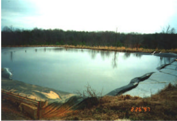
Rainwater accumulation on the previous cover at Martin Farm
