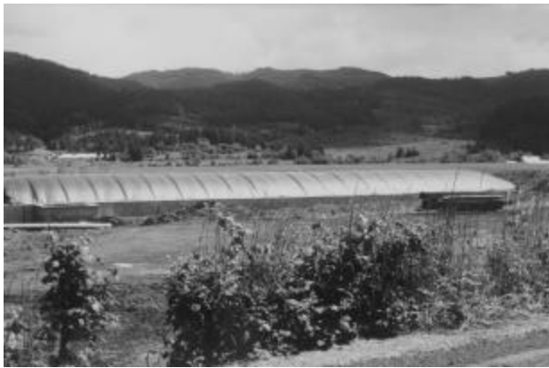
Craven Farms' Plug Flow Digester. The digester is 140 feet long.
