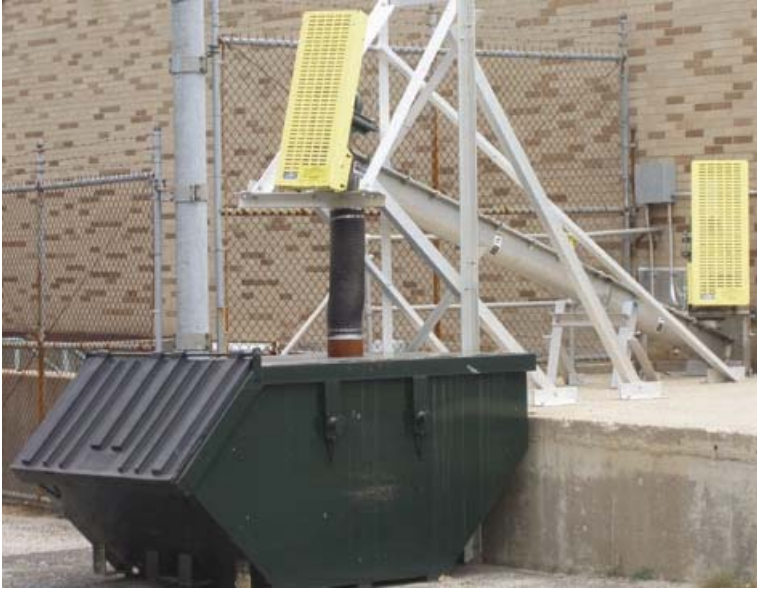
Photograph #3 – Animal bedding screw feed conveyor exiting building and emptying into the dumpster
