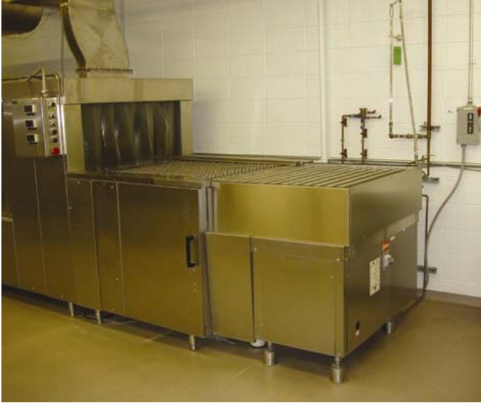
Photograph #1 – Animal cage wash facility with attached animal bedding grinder in the foreground.
