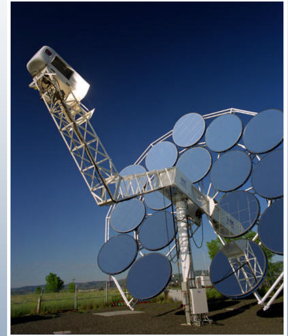
Concentrated Solar Thermal (Stirling engine)
