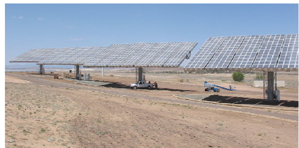
Figure 5. Amonix Inc.'s high-performance concentrator modules in an Arizona Public Service Solar Power Plant. For scale, note white pickup truck beneath the module.
