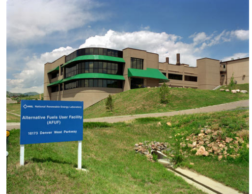
An addition to the Alternative Fuels User Facility will expand the Laboratory's capabilities to develop new cellulosic ethanol technologies.
