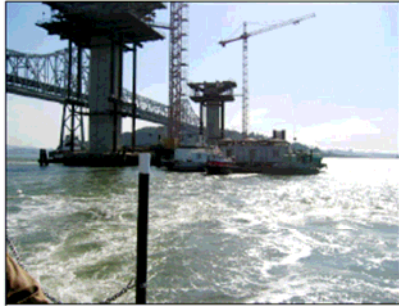
Figure 1: Pier footing at E4W
