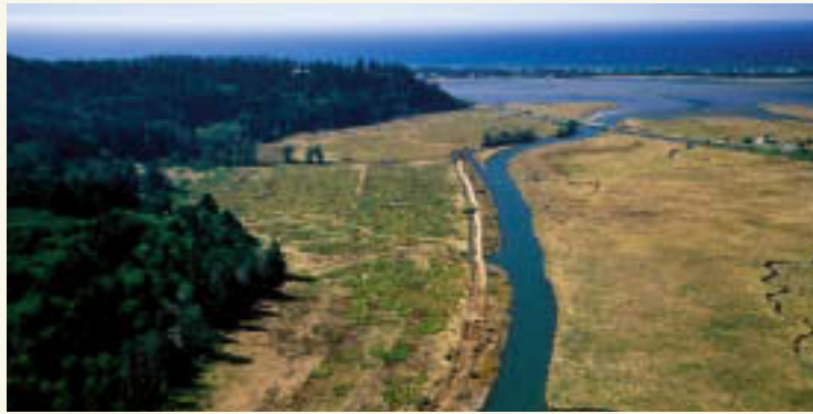
Dike was removed on the left bank of Millport Slough at Oregon Coast NWR Complex. The natural reference marsh is on the right bank. (USFWS)
