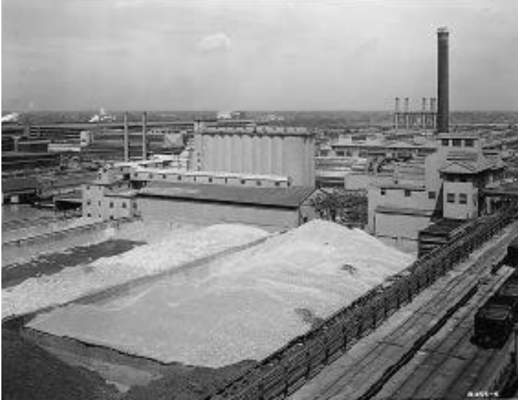
FIG. 6. Ford Rouge Cement Plant, 1945, from the collections of Henry Ford Museum & Greenfield Village and Ford Motor Company
