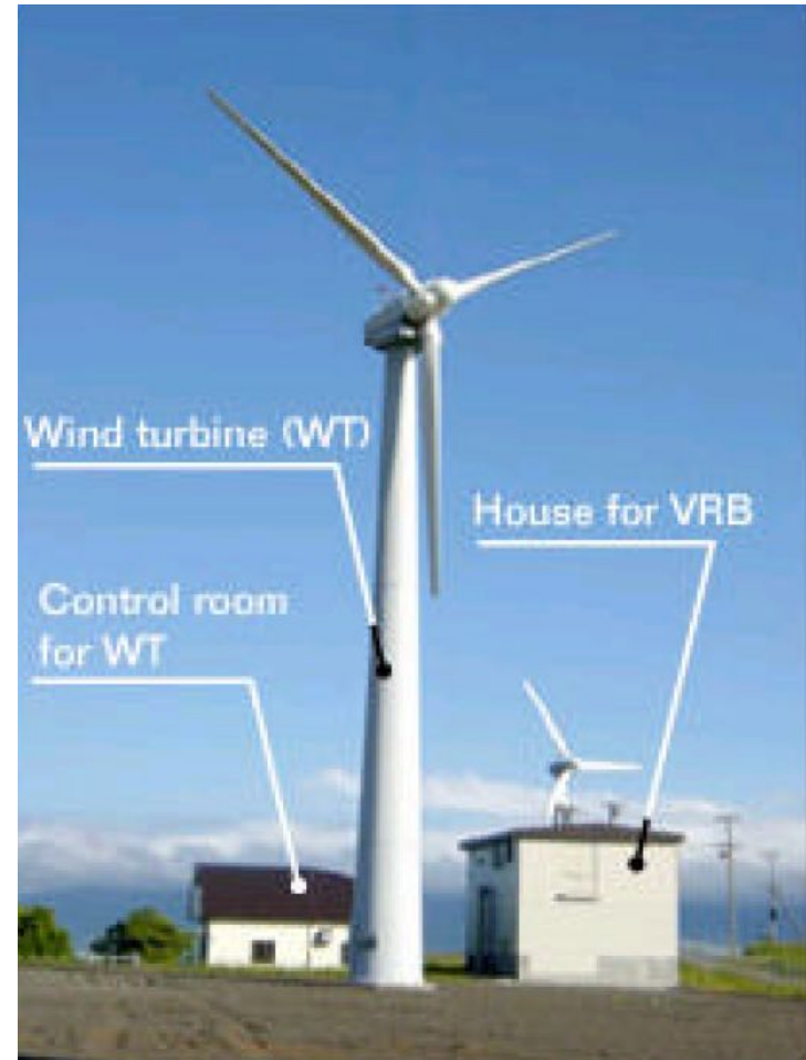
Wind Turbine with Vanadium Redox Flow Battery in Hokkaido, Japan (Courtesy NEDO)
