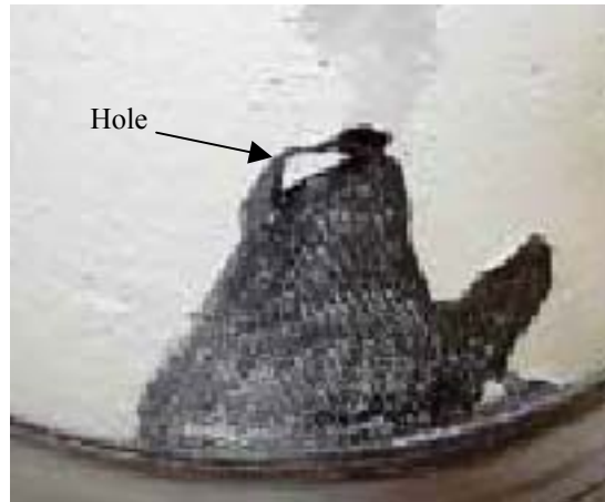
Fig. 5. Hole in an EBC spalled area of the inner liner that formed after 13,937 hours.
