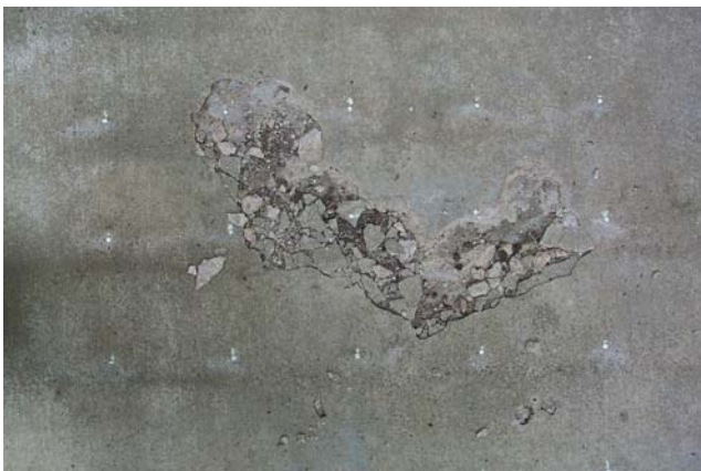
Figure 2.—(a) Concrete damage that has penetrated through to the slab's surface, exposing more-competent material (field of view is 90 cm across). (b) Near-surface damage and aggregate characteristics exposed at edge of slab (penny for scale)
