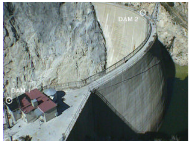
Figure 1. Pacoima Dam. Continuously recording GPS stations DAM1, on the left abutment, and DAM2 at the center of the arch are identified. View is to the north.
