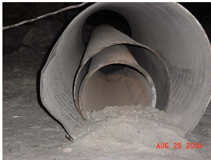
Figure 10: Inside Vent Line 4
