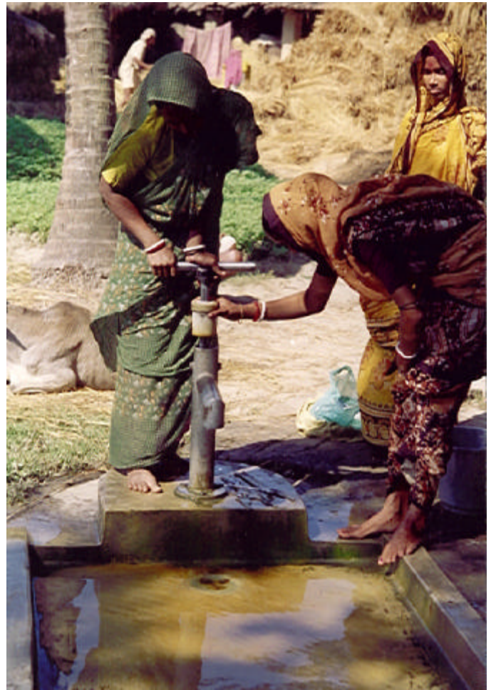
Village women mechanics repair a TARA pump, West Bengal, India. (UNICEF)
