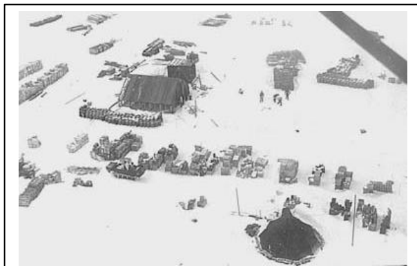
Figure A.4 Maudheim, as seen from the air, under construction. The large structure in the upper left is the first of two huts. Just to the right of this are four men digging the foundation for the second hut.
