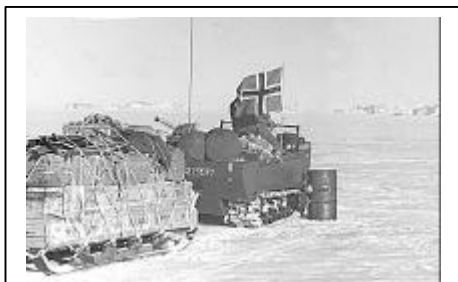
Figure 1.1 NBSX used three tracked amphibious vehicles (Weasels) to transport people and heavy loads of supplies for extended traverses.
