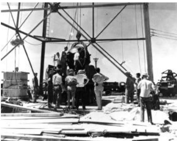
Trinity device being readied. Source: Department of Energy.
