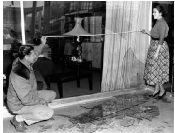
Broken plate glass window in downtown Las Vegas from the Baker-Two shot. Source: AP/Wide World Photos.
