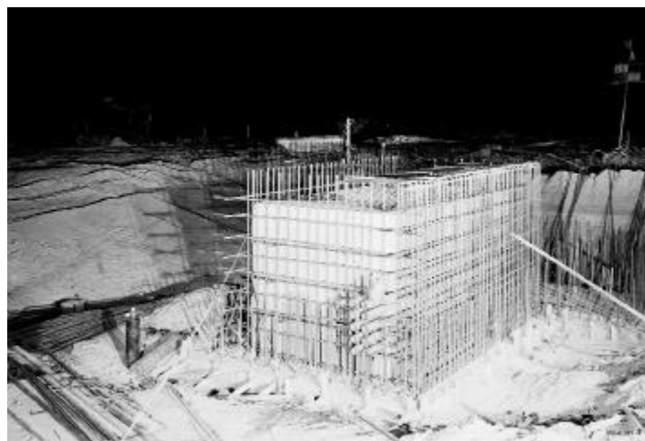
Blockhouse under construction. Source: Los Alamos National Laboratory.
