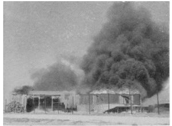
With the completion of Sandstone, temporary structures were torn down and burned. Source: Reprinted from Clarence H. White, ed., Operation Sandstone: The Story of Joint Task Force Seven (Washington: Infantry Journal Press, 1949), p. 64.
