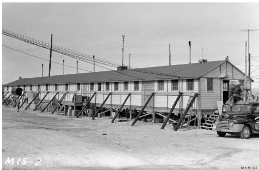
South side of the control point building. Entrance to the control room is at right. Men on porch are looking north toward ground zero. Note braces shoring up the building. Source: Los Alamos National Laboratory.
