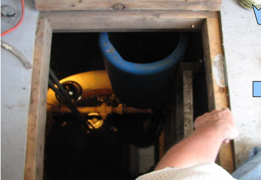
Well with submersed pump that moves ditch water into the shed.
