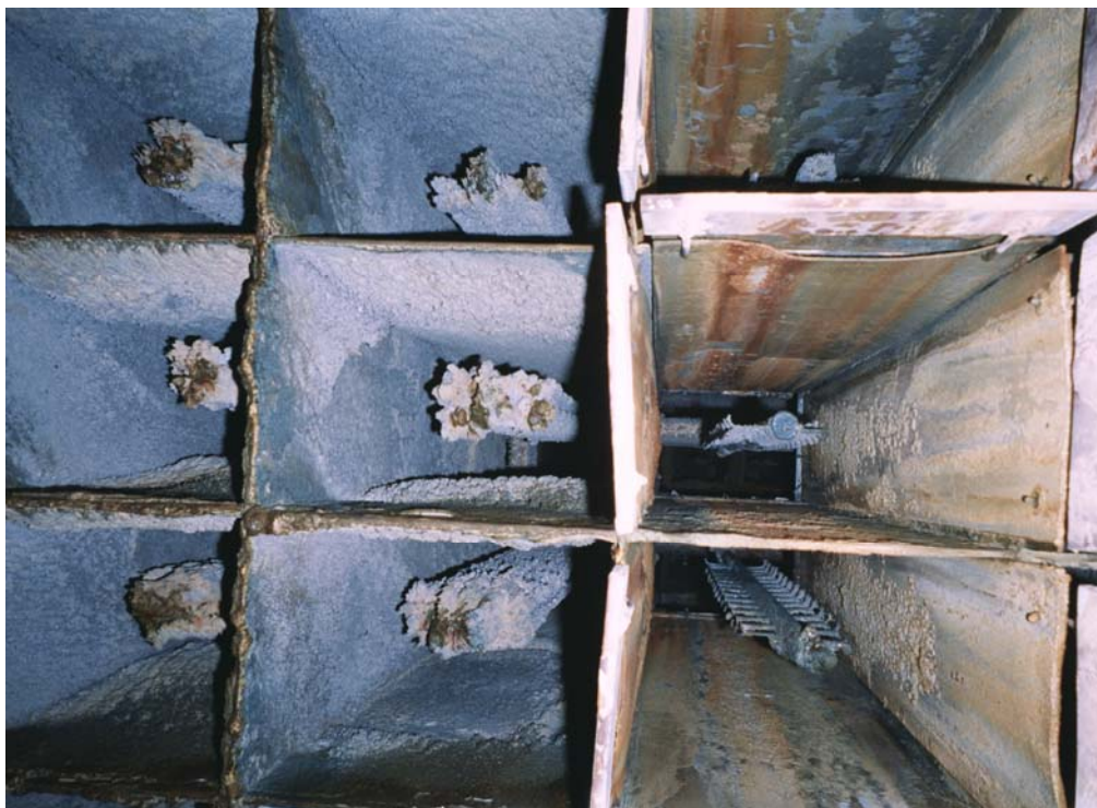
Figure 7: Picture of Membrane Build-up Test
