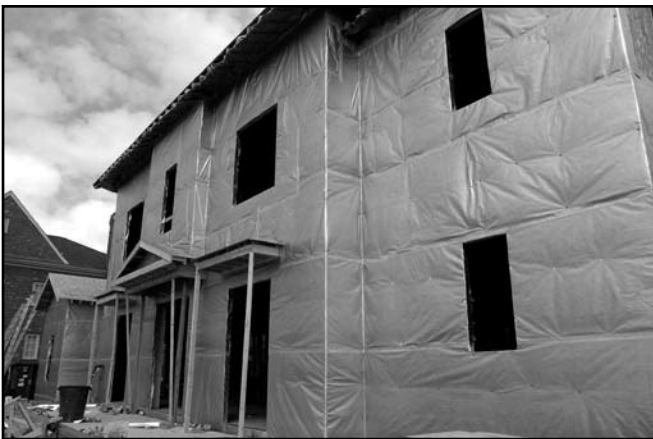
Figure 7. Although DuPont touts Tyvek ThermaWrap as a “low-e” membrane, the emissivity of the product remains a closely guarded secret.
