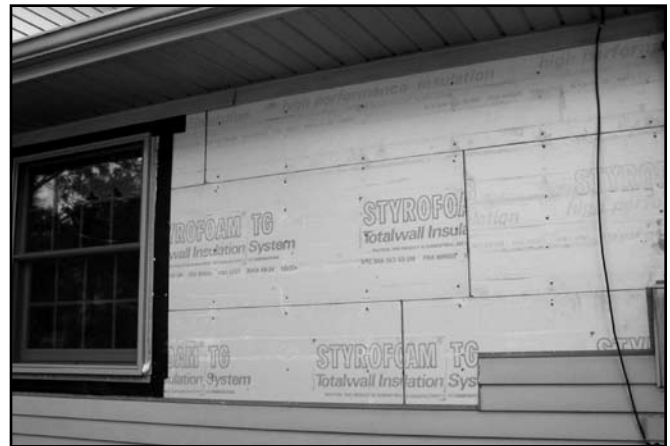
Figure 1. The Dow Styrofoam sheathing on Timothy Lenahan's Ohio house was installed in 1977.
