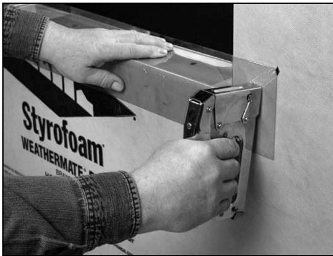
Figure 10. The Dow Weathermate Sill Pan is a thin, transparent flashing that appears to be made of “blister pack” plastic.
