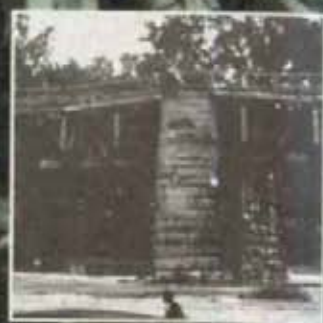
Bolivar aqueduct spanning the Tuscarawas River
