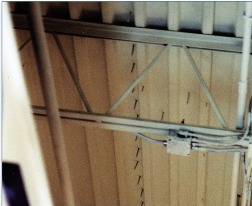
Figure 6-42 View of the underside of a steel deck. The mechanically attached single-ply membrane fastener rows ran parallel to the top flange of the steel deck.
