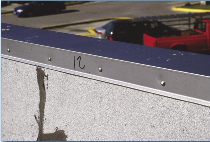
Figure 6-39 This coping was attached with ¼-inch diameter stainless steel concrete spikes at 12 inches on center. When the fastener is placed in wood, #14 stainless steel screws with stainless steel washers are recommended. Also, in the corner areas, the fasteners should be more closely spaced (the spacing will depend upon the design wind loads). ANSI/SPRI ES-1 provides guidance on fastener spacing and thickness of the coping/edge flashing.
