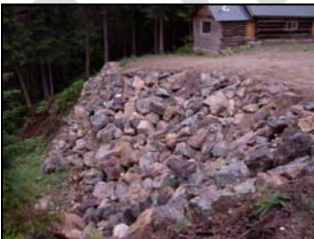
Picture 5. Rock retaining wall north of Cabin.
