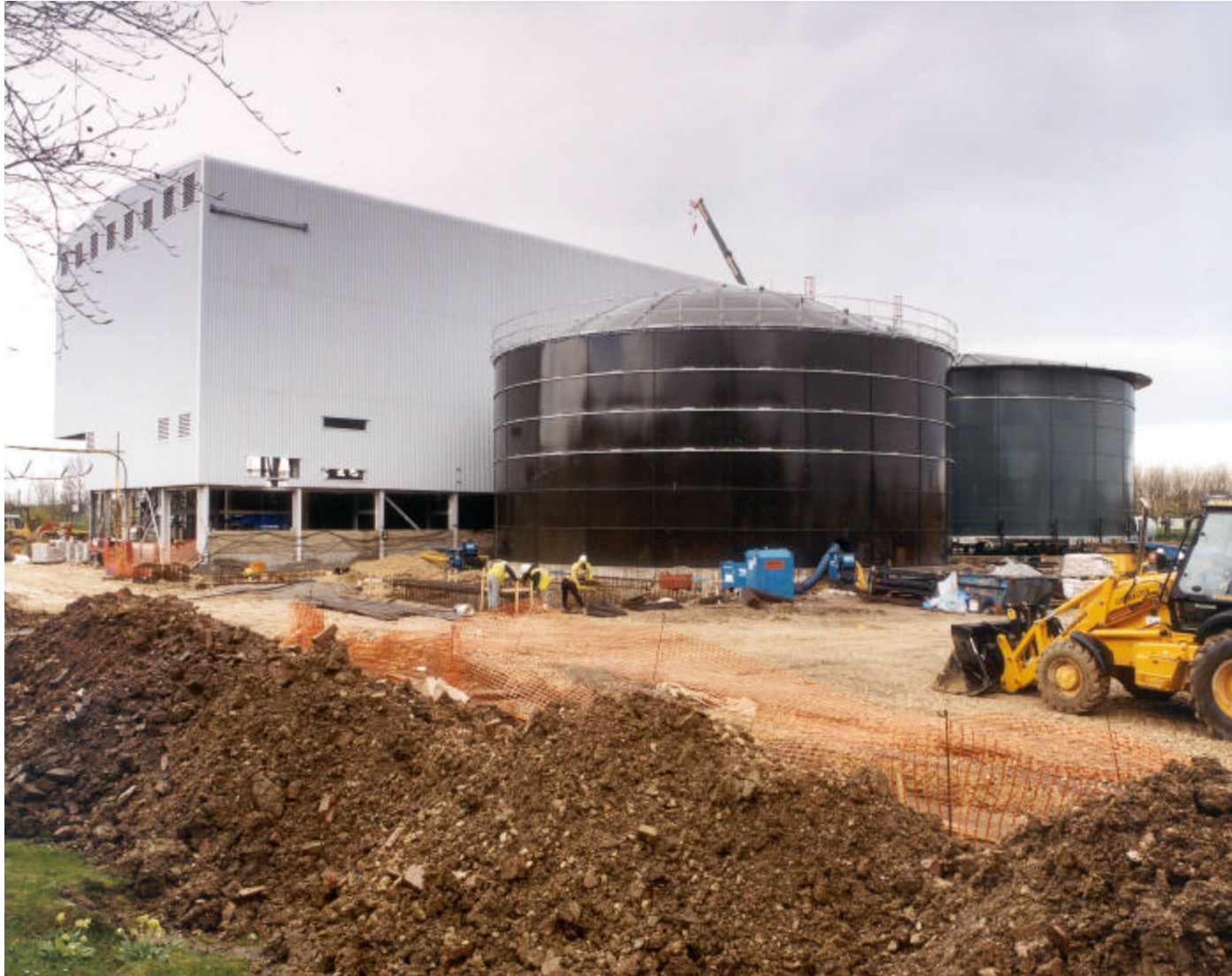
Figure B-1 Current Construction of a Regenesys™ Facility
