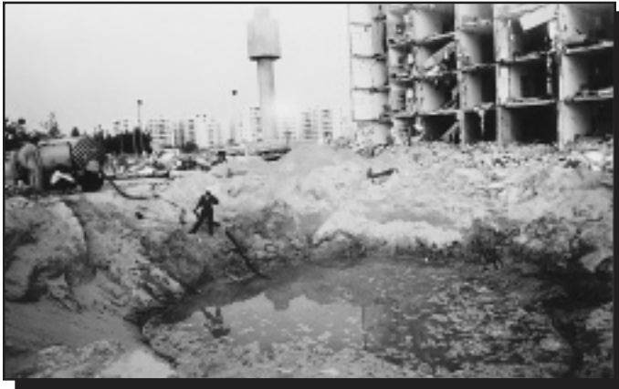
Al-Khobar Towers in Dhahran, Saudi Arabia
