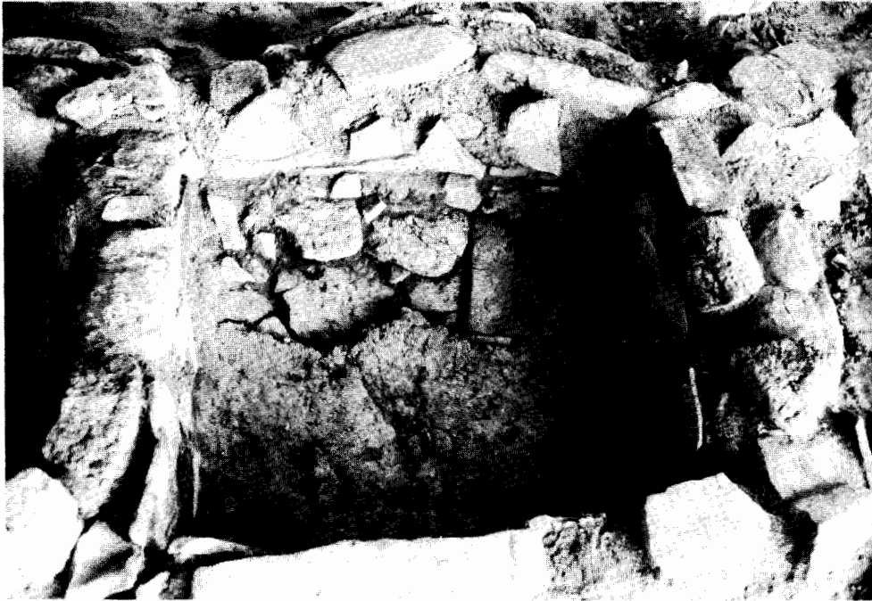
Figure 47. Detail of cleared and stabilized Room A113. Floor stones exposed along southeast wall.
