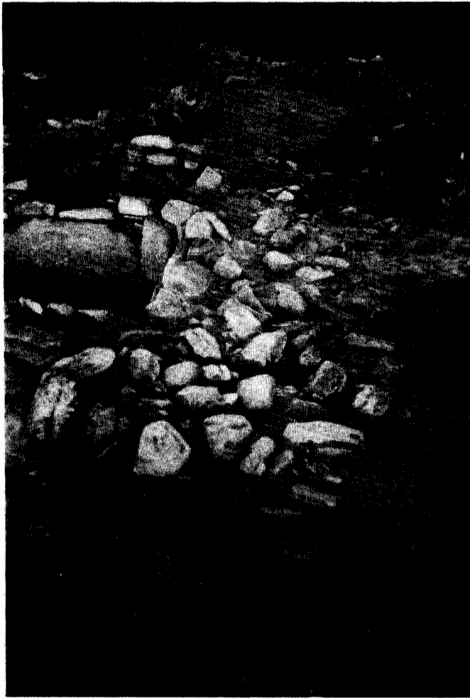
Figure 46. View of exposed wall fall to the northwest of Rooms AI12 and AI13.
