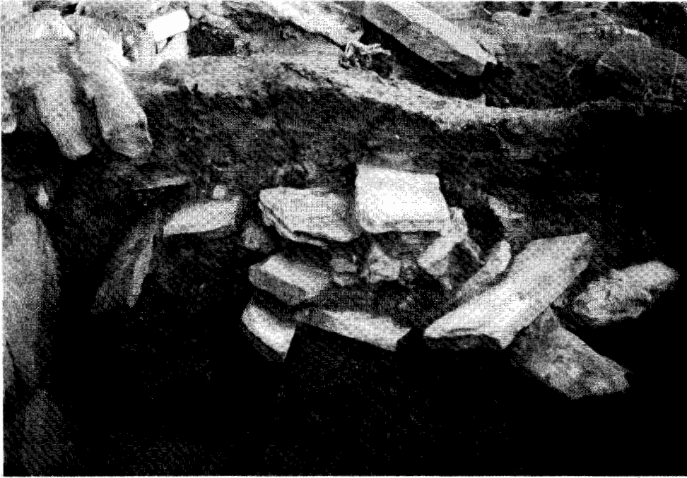
Figure 32. Detail of sectioned-slab building stone in the fill of Room AI6.
