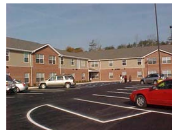
Pictured Above: Knollview Village Apartments, a 48-unit apartment complex for low-income people 55 and older, located on a five-acre knoll just west of St. Albans, at 571 MacCorkle Ave., W, in Charleston, WV. This project was funded through Rural Development's Rural Renting Housing Program.
