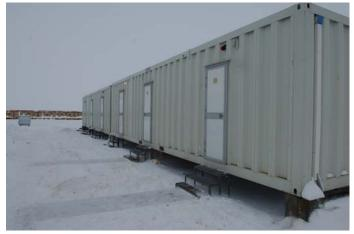
All metal sections used in the structure are subjected to an hot galvanising process (min. 275 g/m<sup>2</sup>). Units can be stacked to form a three-storey high housing complex and can be linked on all four sides.
