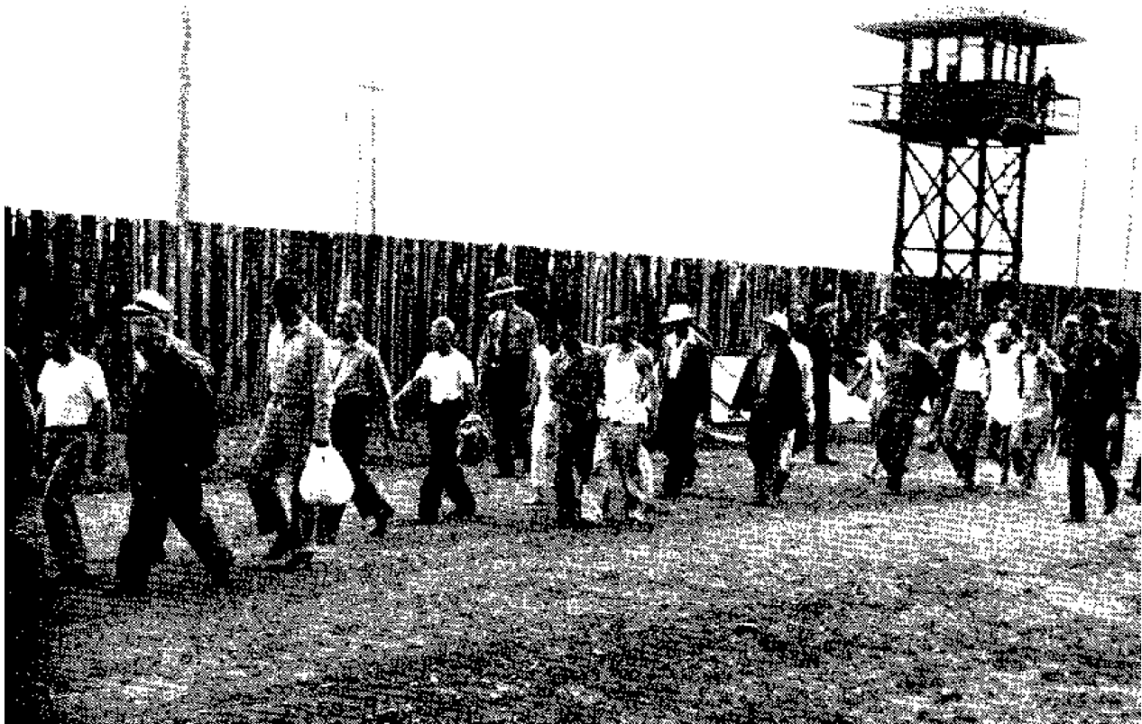
Stockade Tule Lake Segregation Center Newell, Modoc County, California Robert H. Ross, War Relocation Authority, 1944-1946 Historic Photograph 3 of 8
