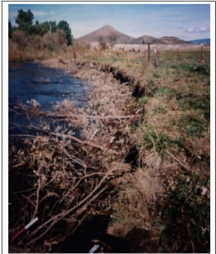
Long vertical bank with matting newly completed.
