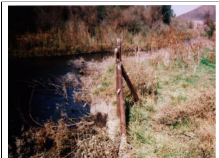
This fence post was 20 feet back from the edge of the stream when installed in 1996.
