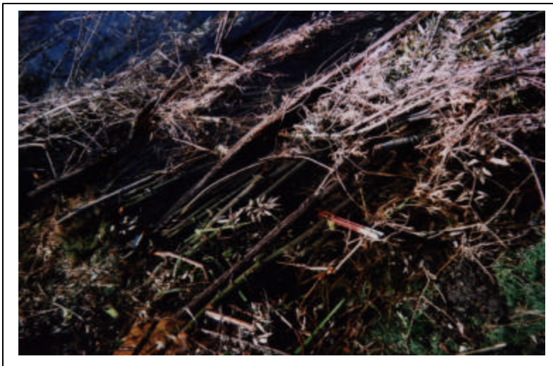
Close-up showing closely spaced willow bundles and bent T posts.
