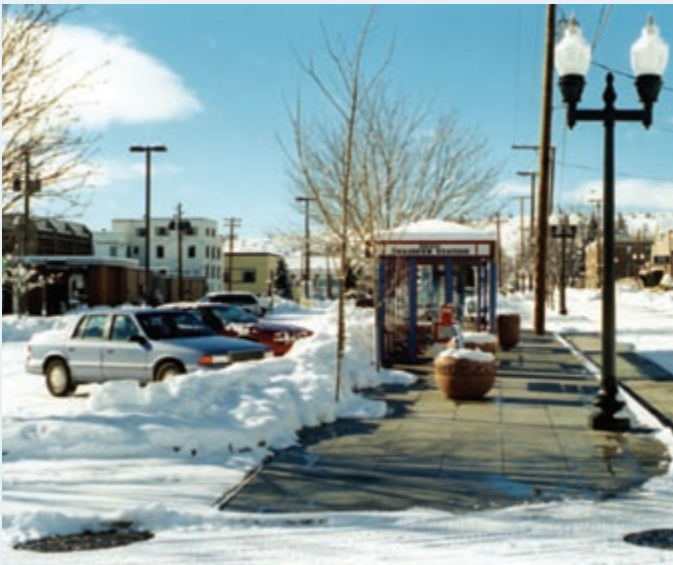
In Klamath Falls, Oregon, the city applies direct-use geothermal for keeping sidewalks and bridges clear and dry after a snowfall.
