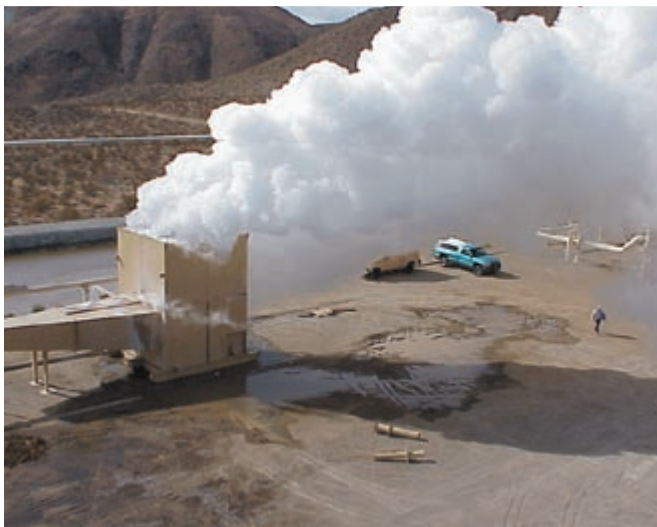
The Low Emissions Atmospheric Metering Separator (LEAMS) helps geothermal well testing achieve “clean energy” status.
