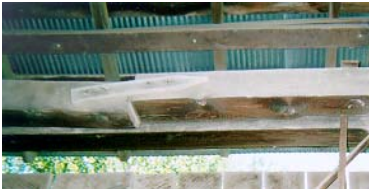
Figure 4. Chambers Road Bridge, detail of butt joint
