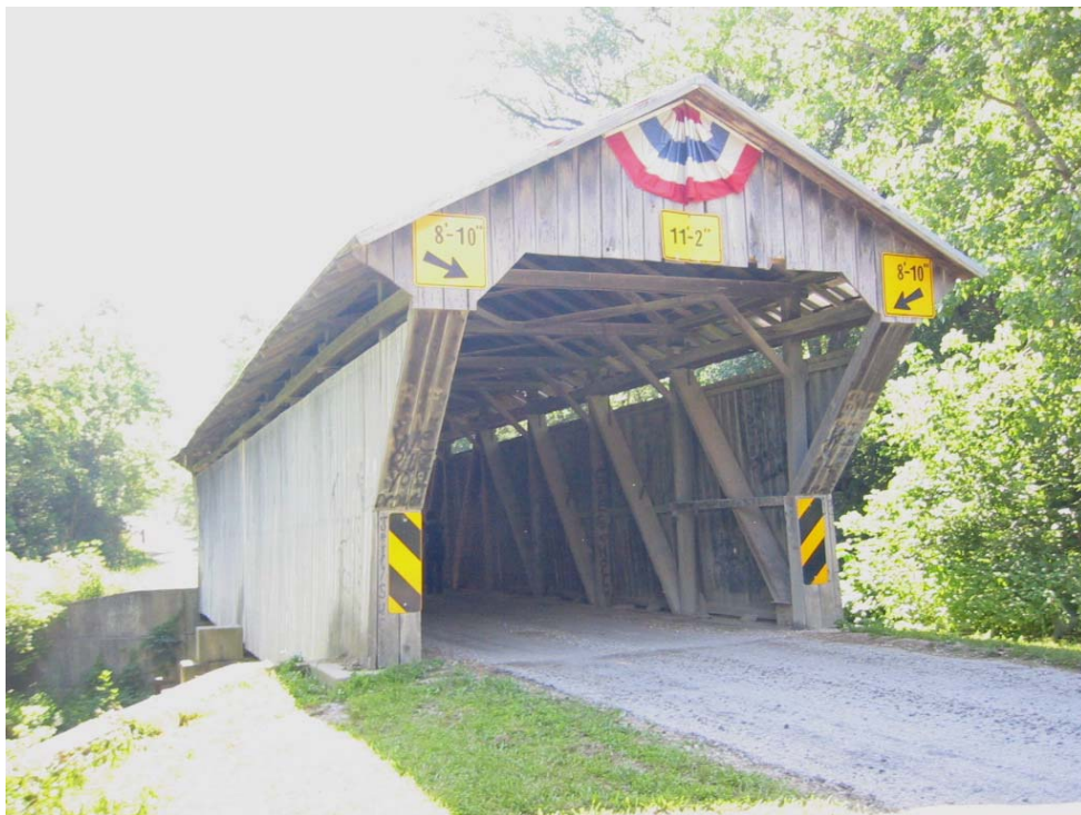
Figure 3. Chambers Road Bridge, built by Everett Sherman in 1883
