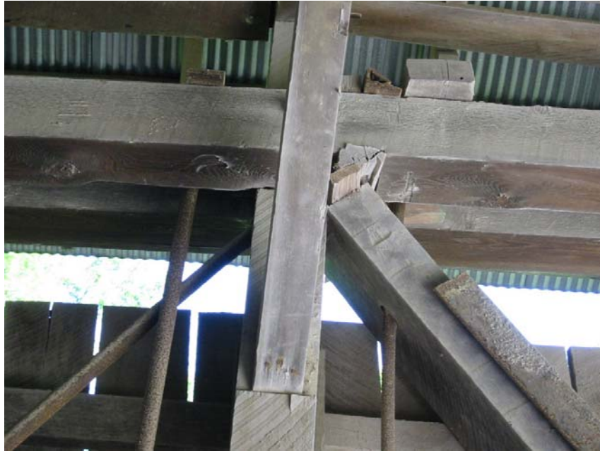
Figure 5. Chambers Road Bridge, detail of connection
