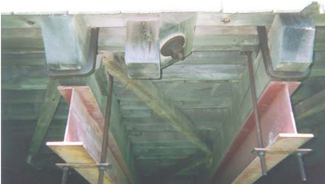
Figure 9. Underside of U-bolt connection showing the retrofitted steel beams
